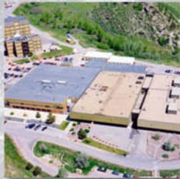
Electronics Mfg Facility
